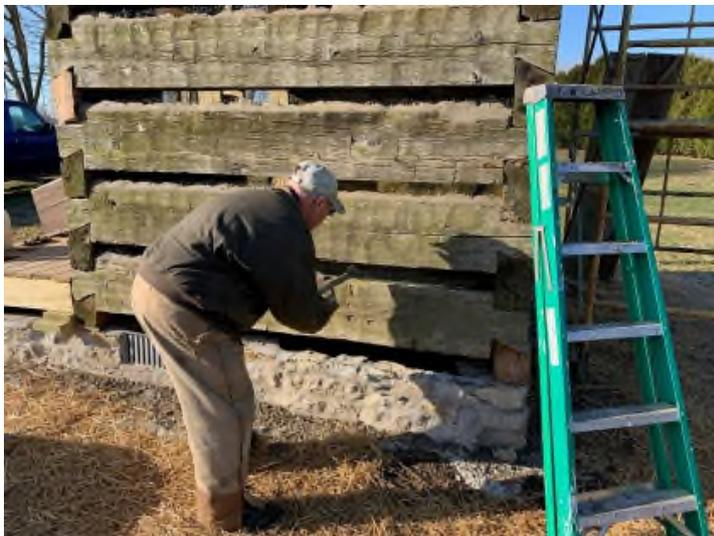
Brice Crowel starts the "chink and gob" operations to close the spaces between the logs and provide weather-tight protection for the Shanty. He is using wire mesh and mortar.
