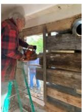
M-W-F crew leader Mac Carlisle shapes the opening in the log wall damaged by the potbelly stove's overheated outlet pipe. Metal webbing between the logs becomes "chink" and will hold the "gob" (like hardened mud) to seal the open space.
