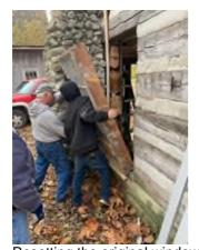
Resetting the original window after the fire damaged logs in the back wall were replaced make this maintenance job almost complete. The Kuns Cabin came to Canal Park from the rural Flora area in the early 1980s as the first of over a dozen buildings moved to Canal. If you would like to volunteer and work with the MWF crew contact admin@canalcenter.org
