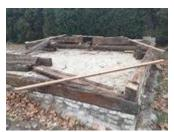
Salvaged squared logs from the old barn near Bringhurst take the form of the outside walls as they come back together on a new footing. Note the notched corner to see how these logs are held together and form a solid wall above the stone foundation.
