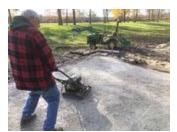
Here Mac Carlisle is firming the crushed stone floor inside the finished foundation made of those limestone chunks mortored in place. This compactor was recently donated by contractor Jack Cohee as he is retiring from his construction business.
