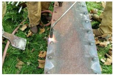
Our M-W-F crew has been busy throughout the summer and fall with metal repairs and painting of completed bridge parts. Here, we heat with a torch the zone between rivets and prepare to pound out the "pack rust" that has accumulated between the flat plate and the side rails of this upper chord member. Pack rust accumulates as the bridge ages and eventually buckles the plate.
