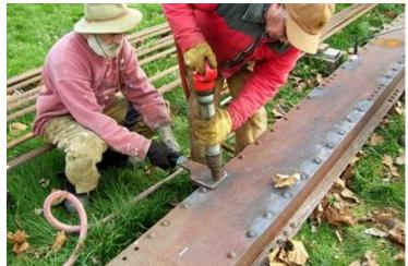
Immediately after heating the space between the rivets the M-W-F crew hammers down the bulge. Note the lighter gray color across from the row of rivets where that side had already been heated and hammered to drive out the rust. This action takes time, lots of crew effort, and sometimes even sweat in the heat of last summer.
