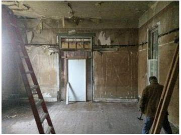
The inside of this small church had walls that were plastered and a raised area at the back where the minister would conduct his services. The floor was remarkably sturdy and refinishable. The front door had been replaced with a more modern door but the window transome above was covered on the outside. We will restore all this to its original looks.
