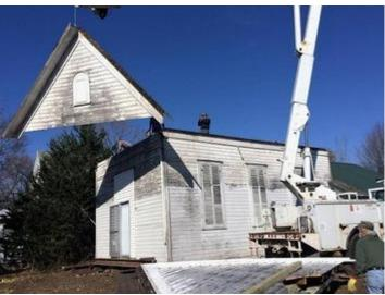
Preparing for the move took contractor Waylan Graybill and his crew to the heights and by removing rafters and gable ends the plan was to allow clearance for overhead wire and tree limbs during its travel down residential streets.
