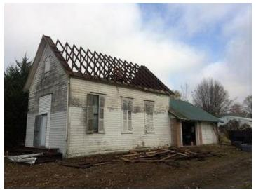
Roof removed and now down to the rafters the moving contractor begins his preparation for the move. Shutters on the windows are in good shape and Mr. Treece wanted us to save the garage at the back for his later use.
