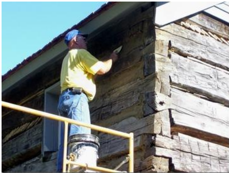
Dave Smith places mortar on the spaces of the second floor.
