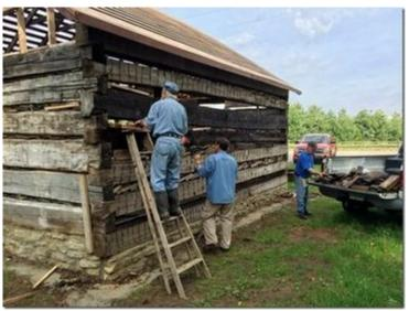
Busy as bees, the M-W-F crew places cedar shingles on the roof and chinks the space between logs. Next will be the placing of "gob" (mortar) to complete the weatherizing before it can be used as the Loom House.
