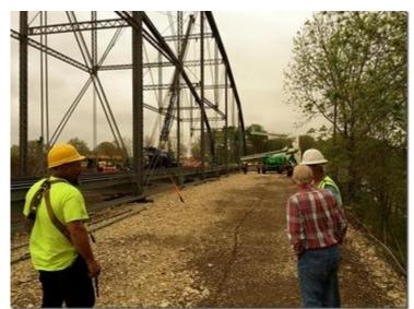
Too big for our M-W-F crew is the 300 foot long bridge from Freedom, Indiana. Contractors for the City of Delphi and INDOT are reassembling this span to become the pedestrian crossing over the new four lane Hoosier Heartland Highway. The trail and span follow the old railbed east a mile to finally encounter the Monon High Bridge over Deer Creek.
