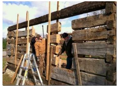
As logs allow, we find locations for windows and doors. A modern chain saw now makes this cutting easier but we all try to imagine how the old-timers would have done it. The setting for this building is near the parking lot and will be the home of several looms that the Canal has.
