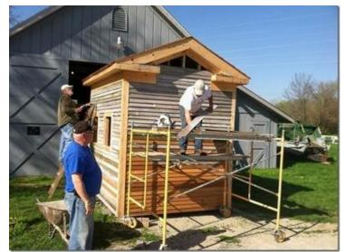
Last month the M-W-F crew built the frame and placed cedar shingles on the replica Mill building, another hand-crafted interpretive exhibit for Canal Park. This model will be placed on a site near the boat warehouse in the Red Bridge Settlement. It will have an mill wheel that operates to give the illusion of how mills were powered by water.
