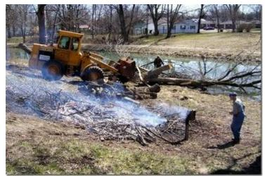
Several large trees along the canal bank had to be cleared to make way for the placement of the Gray Bridge later this summer. The foundation "footer" for one end of the bridge will be located near where this burning brush pile is. In the meantime, the M-W-F crew continues to work on repairing, cleaning and painting individual pieces of the steel bridge.
