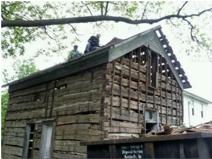
In May our M-W-F crew began disassembly of this rural Burrows area log house. Donor Jim Mullin from Georgia has allowed us to come and take apart this well preserved story and a half building. We intend to restore it and place the building in Canal Park, perhaps starting later this year.
