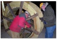
Brice Crowel (with drill) and Al Auffart are building the Mill wheel's catchment cavities. The Mill exhibit will be placed in Red Bridge Settlement and will have a water source to actually turn the wheel.
