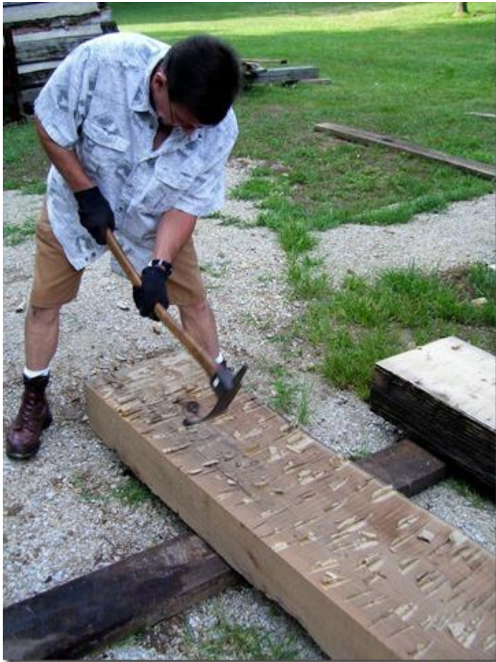
Clay Sledd chips away at the sawed side of an old timber to make it look more like an ax had been used to cut it. This side will be seen from the inside of the log house.
