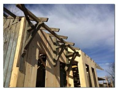
Railroad style "corbels" extend the length of the roof to provide rain protection for persons waiting on boarding trains. This design is typical of depots where standard plans were adopted by all railroads. They only changed slightly about every decade. This Erie Lackawanna station depot was built in 1884 at Leiters Ford.
