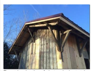
The metal overlaps the roof edge to seal and protect the building. New vertical  $1 \times 12$  pine boards will be accented with "batten" to make the siding look like the original. Some of the original 1884 boards are still good and will be stripped of old paint and spray painted when the project is completed. New windows will be secured
