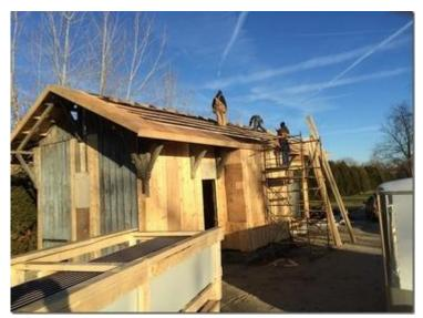
Finally on Christmas Eve day a crew of roofers coordinated by Wylan Graybill were preparing to install "standing seam" metal roofing. They placed sheets of plywood showing board like grooves under the roof at the corbel extensions to appear like the original railroad design.
