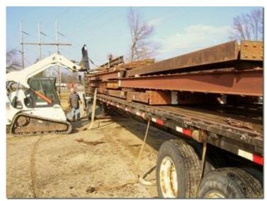
On Friday, the contractor's crew from Greencastle brought the disassembled iron bridge to Canal Park. Four semi truckloads were placed on the ground on blocking so the volunteer crew can begin picking a "piece at a time" and working on cleaning, restoring and
