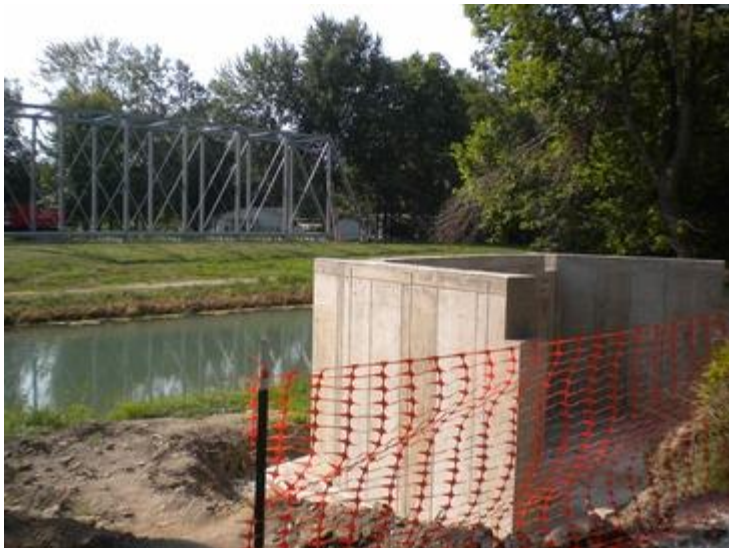
Fast forward a week or more, and now the west side abutment is done, and the east side abutment has been poured. You'll notice the bridge in the background, across the canal. Be sure to check our Facebook page for new photos as we move toward completion of this project!
